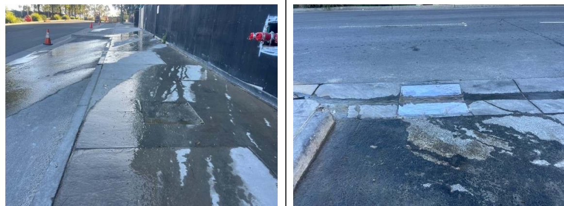
Photos 7 & 8: Seepage was observed from under the hoarding along De Clambe Drive. A leak was detected at the time of the audit and managed.
