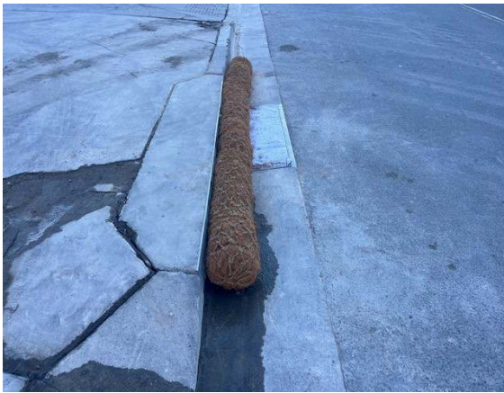
Photo 9: Controls in place on stormwater inlets
