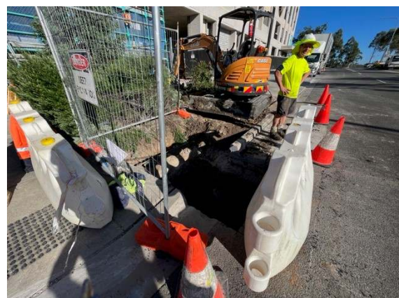
Photos 15&16: Pedestrian diversion signage place on the corner of Andalusian Way and Mandala Drive for stormwater connection works
