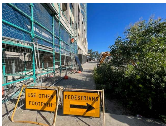
Photos 15&16: Pedestrian diversion signage place on the corner of Andalusian Way and Mandala Drive for stormwater connection works
